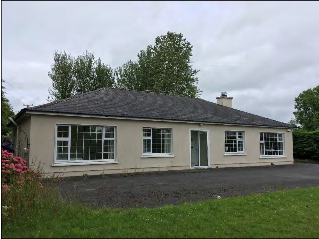
Plate 4-2 Dwelling house to be demolished at Gortnaloura, classified as Buildings and Artificial Surfaces (BL3)
